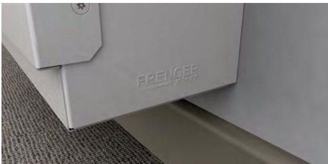
Wall Mounted Armis LST Radiator Cover Detail
