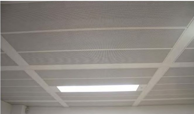
Hook-on Chilled Ceiling Tile Installation
