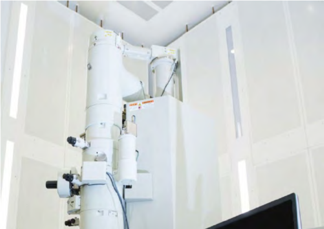
Wall Mounted Chilled Tile Installation
