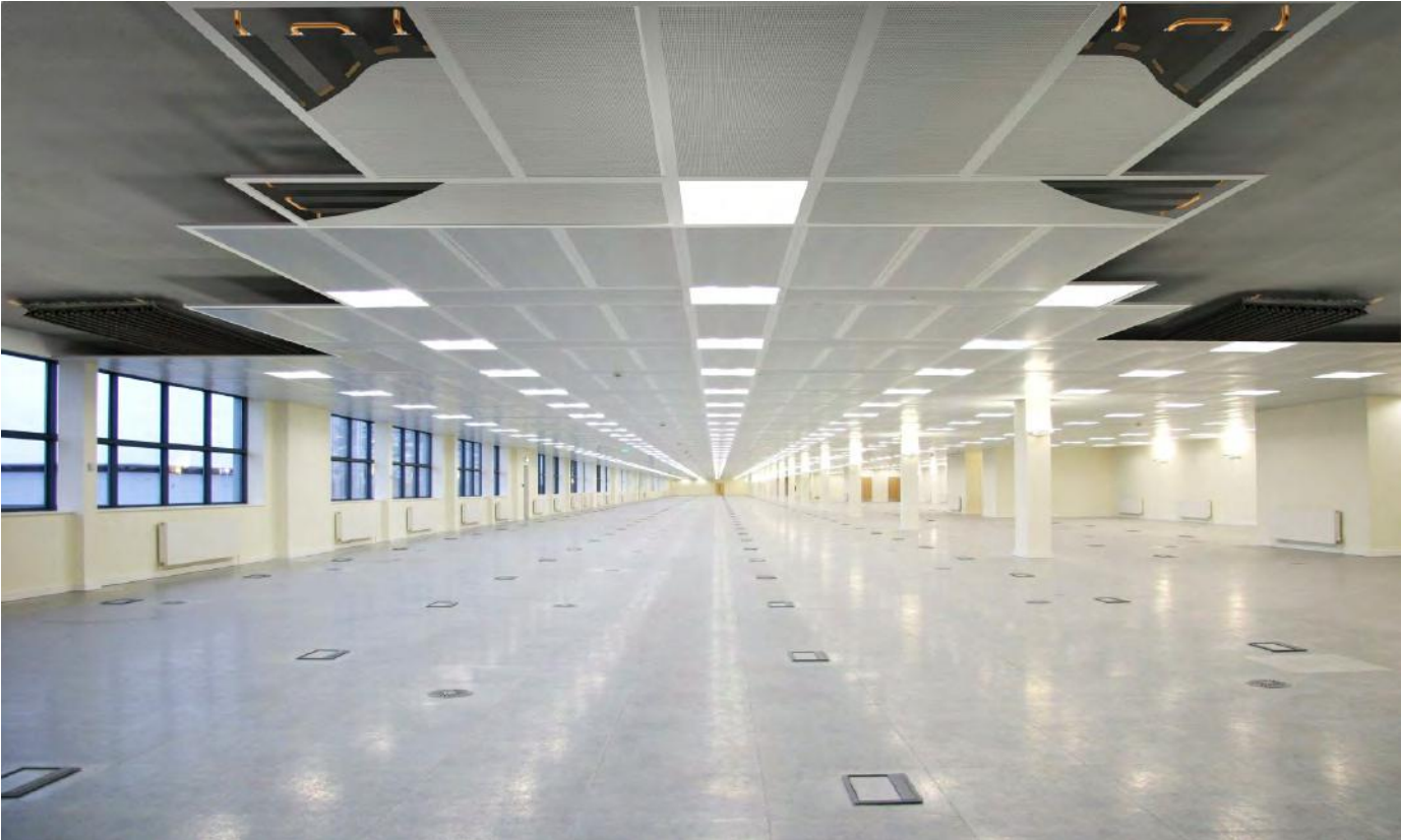
Concealed Radiant Chilled Beams Note: The perimeter ceiling tile perforations are the same size and percentage open areas as (Micro perf) the core zones with traditional chilled ceiling tiles.
