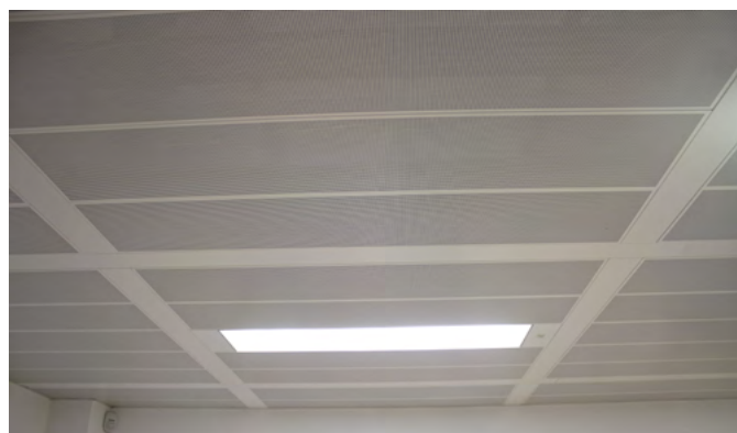
Hook-on Chilled Ceiling Tile Installation
