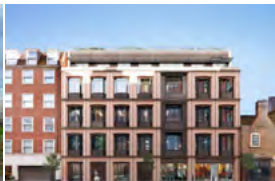
18-20 Grosvenor Street London, UK - 2014 Active Chilled Beams
