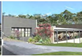
Kingston Aged Care Australia - 2009 Active Chilled Beams
