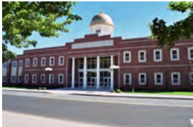
Ocean City School New Jersey, USA - 2015 Active Chilled Beams
