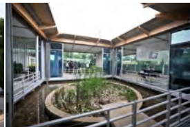
Vodafone Innovation South Africa - 2011 Passive Chilled Beams
