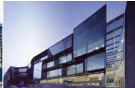
IMAS Hobart Australia - 2012 Passive Chilled Beams
