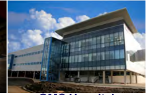
QMC Hospital Nottingham, UK - 2008 Active Chilled Beams
