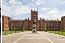
Queens University Belfast, UK - 2015 Passive Chilled Beams
