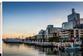
King Street Wharf Australia - 2008 Passive Chilled Beams
