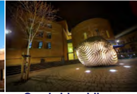
Cambridge Library Cambridge, UK - 2008 Active Chilled Beams
