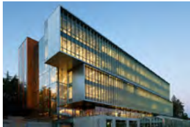
UW Life Sciences Seattle, USA - 2017 Passive Chilled Beams
