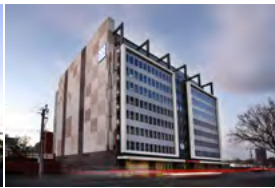
South Australia Police Adelaide, Australia - 2009 Passive Chilled Beams
