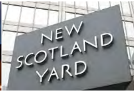
New Scotland Yard London, UK - 2010 Passive Chilled Beams
