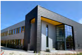
NTU Engineering Nottingham, UK - 2019 Multiservice Radiant Panels
