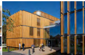
Alder Hay Research & Education Liverpool, UK - 2014 Active Chilled Beams
