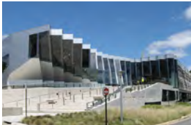
ANU Australia - 2013 Active Chilled Beams
