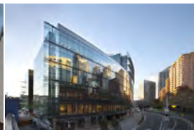
Kangan Batman Tafe Australia - 2010 Active & Passive Chilled Beams
