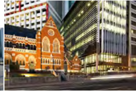
Wesley House Brisbane, Australia - 2008 Passive Chilled Beams
