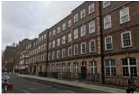
LSTM London, UK - 2022 Active Chilled Beams
