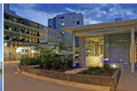
Royal Hobart Hospital Hobart, Tasmania - 2010 Active Chilled Beams
