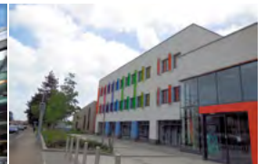
Northbrook College Worthing, UK - 2014 Active Multiservice
