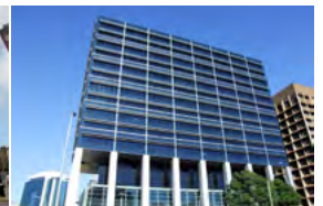
Sydney Water House Australia - 2008 Passive Chilled Beams
