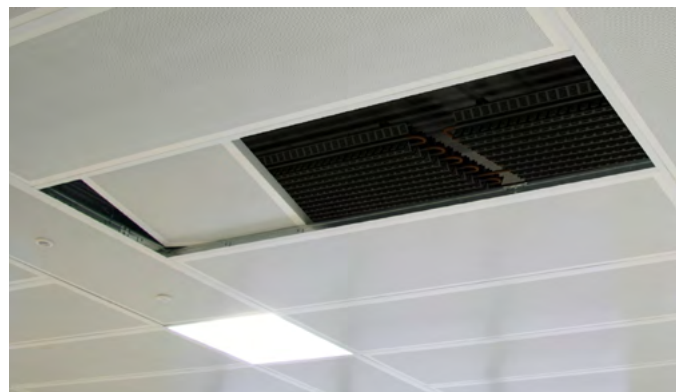
“Hybrid” Radiant / Convective Chilled Beam Ceiling
