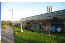
Exeter University Exeter, UK - 2012 Active Chilled Beams
