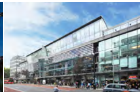
High Holborn London, UK - 2014 Active Multiservice / Active Chilled Beams
