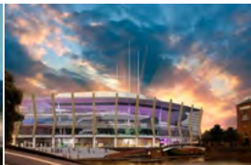
Arena Birmingham Birmingham, UK - 2014 Passive Chilled Beams
