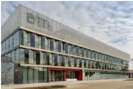
Brunel University London, UK - 2017 Active & Passive Chilled Beams
