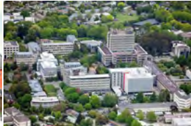
Uni of Canterbury New Zealand - 2016 Active Chilled Beams
