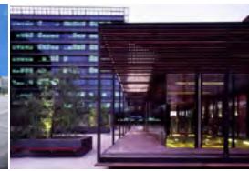
Parramatta Justice Sydney, Australia - 2006 Passive Chilled Beams
