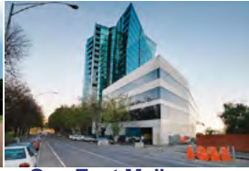
One East Melbourne Victoria, Australia - 2008 Passive Chilled Beams
