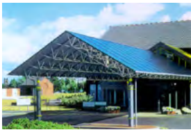
Wrexham A&E Wrexham, UK - 2008 Active Chilled Beams
