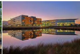
Wollongong University NSW, Australia - 2011 Passive Chilled Beams
