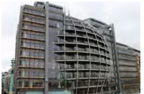
Ofcom Riverside House London, UK - 2018 Passive Multiservice
