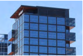
Hub on Causeway Boston, US - 2022 Active Chilled Beams
