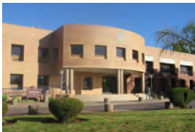
University of Botswana Botswana - 2011 Active Chilled Beams
