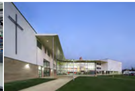
All Saints Academy Cheltenham, UK - 2011 Passive Chilled Beams
