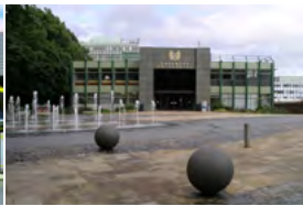
Coventry University Coventry, UK - 2008 Active Chilled Beams
