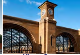
Kings Cross London, UK - 2008 Active Chilled Beams
