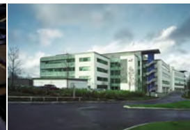
BT Leavesden Watford, UK - 2002 Passive Chilled Beams
