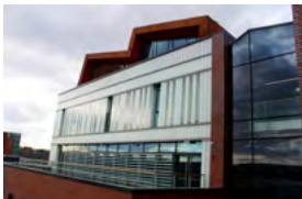
Charles Street, Sheffield University Sheffield, UK - 2015 Passive Chilled Beams
