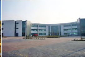
Business Centre Liverpool, UK - 2008 Active Chilled Beams
