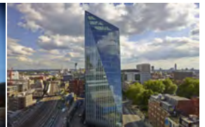
240 Blackfriars Road London, UK - 2014 Active Chilled Beams
