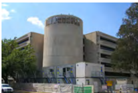
Edmund Barton Canberra, Australia - 2009 Active Chilled Beams
