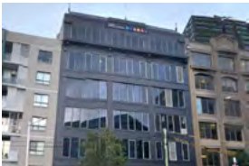
SAE Qantm Sydney, Australia - 2016 Passive Chilled Beams
