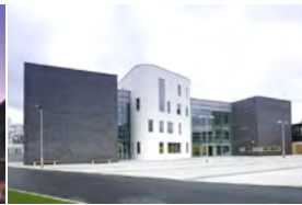
Loxford School London, UK - 2009 Active Chilled Beams
