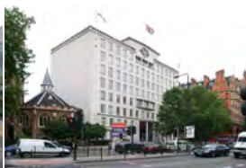
Woolworth House London, UK - 2003 Active Multiservice
