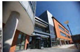
West Suffolk House Ipswich, UK - 2014 Passive Chilled Beams
