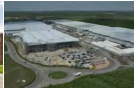
Sports Direct Head Office Derby, UK - 2015 Active Chilled Beams
