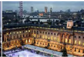
Kings College London, UK - 2009 Passive Chilled Beams
