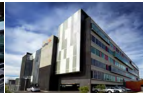
World Park Adelaide, Australia - 2011 Passive Chilled Beams
