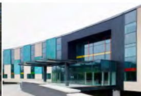
ACAD Hospitals - Stobhill Glasgow, UK - 2008 Active Chilled Beams
