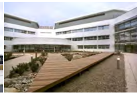
Cheshire Police Cheshire, UK - 2009 Active Chilled Beams
