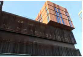
Victorian Heart Hospital Melbourne, AUS - 2021 Active Chilled Beams
