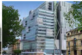
City Centre Tower 8 Australia - 2011 Passive Chilled Beams
