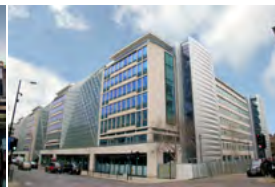
55 Baker Street London, UK - 2008 Active Multiservice
