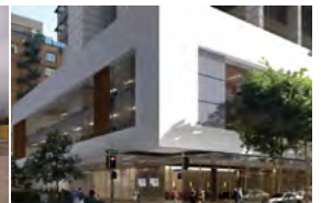
123 Albert Street Brisbane, Australia - 2010 Passive Chilled Beams
