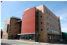
Liverpool College Liverpool, UK - 2010 Active Chilled Beams
