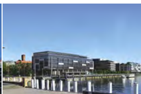
Google Headoffice Sydney, Australia - 2010 Passive Chilled Beams
