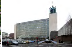
Newcastle Civic Centre Newcastle, UK - 2016 Active Chilled Beams
