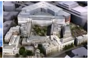
St Barts Hospital London, UK - 2009 Active Chilled Beams
