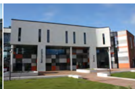
Stafford College Stafford, UK - 2012 Active Chilled Beams
