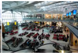
Gatwick Terminal London, UK - 2008 Passive Chilled Beams
