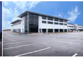
Project Vauxhall UK - 2006 Passive Chilled Beams
