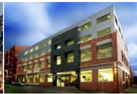
Batman Street Australia - 2009 Passive Chilled Beams
