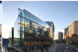
Common Wealth Bank Australia, Sydney - 2012 Passive Chilled Beams
