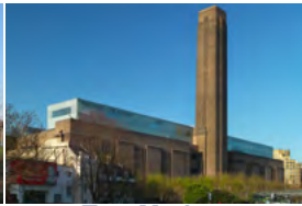
Tate Modern London, UK - 2012 Passive Chilled Beams
