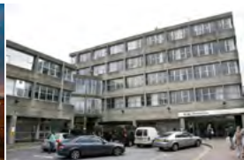
Northwick Park Hospital Harrow, UK - 2014 Active Chilled Beams
