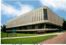
Hallward Library Nottingham, UK - 2008 Active Multiservice
