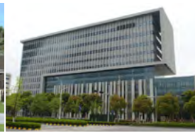
Monash University Australia - 2009 Active Chilled Beams
