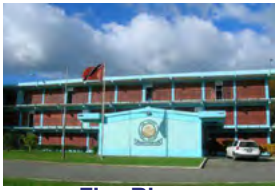
Five Rivers Trinidad - 2010 Passive Chilled Beams
