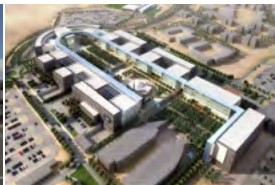
King Saud Bin Abdul Saudi Arabia - 2011 Active Chilled Beams
