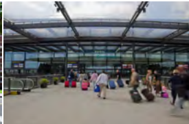
Gatwick Airport Gatwick, UK - 2015 Passive Chilled Beams
