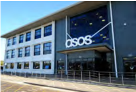
ASOS Leavesden Watford, UK - 2017 Active Chilled Beams
