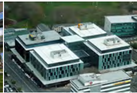
Telcom Square New Zealand - 2010 Passive Chilled Beams
