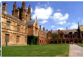
University of Sydney Sydney, Australia - 2007 Passive Chilled Beams
