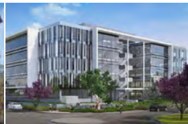
1 Canberra Avenue Australia - 2013 Passive Chilled Beams
