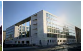
SIEC Tonsley House Australia - 2013 Active & Passive Chilled Beams
