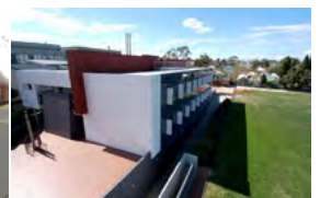
Trinity Grammar Australia - 2012 Passive Chilled Beams
