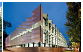
Belconnen Police Australia - 2010 Passive Chilled Beams
