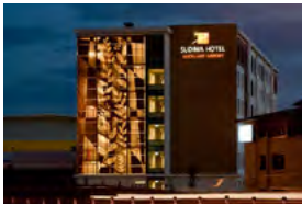
Sudima Hotel New Zealand - 2010 Active Chilled Beams
