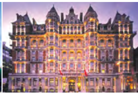
Knightsbridge Hotel London, UK - 2010 Passive Chilled Beams
