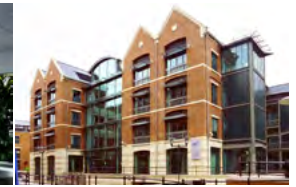
BT Nottingham Nottingham, UK - 1998 Passive Chilled Beams
