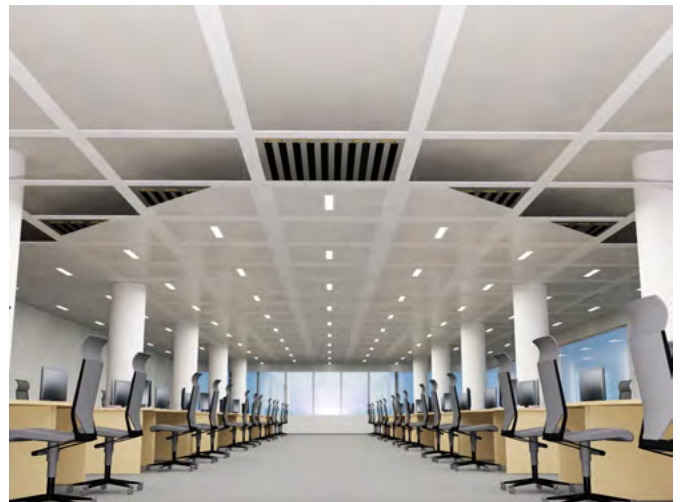
Tartan Grid Ceiling
