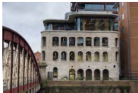
Riverside House Salford, UK - 2019 Passive Chilled Beams
