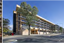
64 Allara Street Australia - 2007 Passive Chilled Beams
