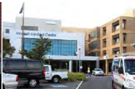
Monash Children's Hospital Australia - 2014 Active Chilled Beams
