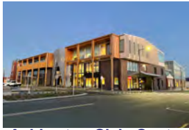
Ashburton Civic Centre Ashburton, NZ - 2023 Active Chilled Beams
