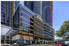
Barangaroo C2 Sydney, Australia - 2016 Passive Chilled Beams
