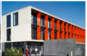
National Film & TV School Beaconsfield, UK - 2016 Active Multiservice / Active Chilled Beams
