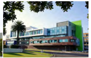
Warnambool Hospital Australia - 2009 Active Chilled Beams
