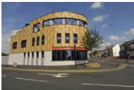
Walthamstow Station Walthamstow, UK - 2011 Passive Chilled Beams
