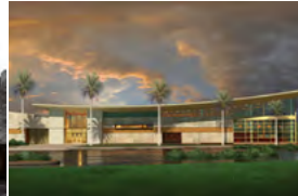
Skyline Hills Library San Diego, USA - 2016 Active Chilled Beams
