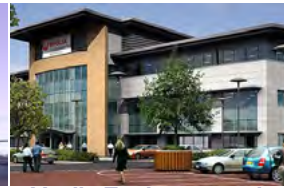
Veolia Environmental Cannock, UK - 2012 Passive Chilled Beams
