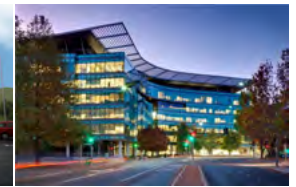
London Circuit Canberra, Australia - 2006 Passive Chilled Beams
