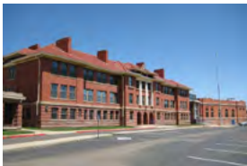
Trinidad School Trinidad & Tobago - 2011 Passive Chilled Beams
