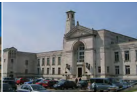
Civic Offices Southampton, UK - 2009 Active Chilled Beams
