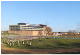
Cambridge Metallurgy Cambridge, UK - 2012 Passive Chilled Beams
