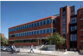
Three Haddington Buildings Dublin, Ireland - 2019 Active Multiservice
