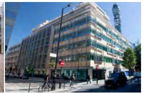
New Cavendish Street London, UK - 2009 Active Multiservice
