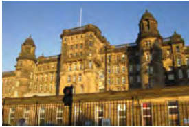
GRI Gynae Glasgow, UK - 2008 Active Chilled Beams
