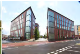
Langley Point Birmingham, UK - 2012 Passive Chilled Beams
