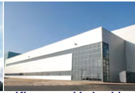
Kingswood Lakeside Cannock, UK - 2010 Passive Chilled Beams
