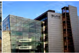
Suffolk County Council Suffolk, UK - 2008 Passive Chilled Beams
