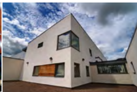
Macmillan Renton Unit Hereford, UK - 2010 Active Chilled Beams
