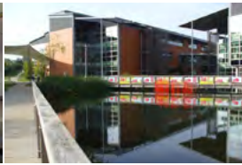
Vodafone London, UK - 2001 Passive Chilled Beams
