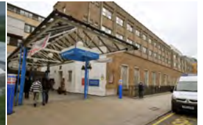
Great Ormond Street Hospital London, UK - 2015 Active Chilled Beams
