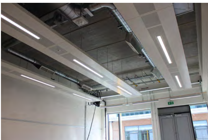
Nottingham Trent University, Engineering Building
