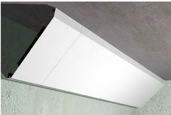
5. Apply NOMS approved non-pickable sealant to all exposed gaps that may be created due to building tolerances.
