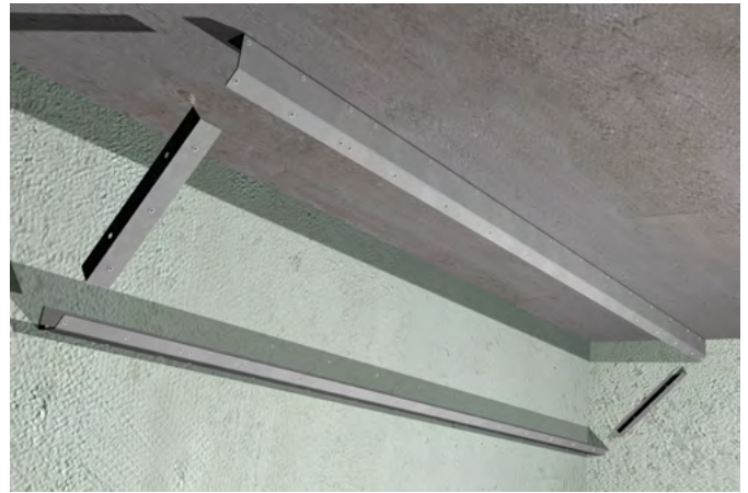
2. Install purpose made 'cut-to-length' ceiling mounting rails and end support rails at the required centers. Ensure rails are level and true to ensure secure panel interconnections.
