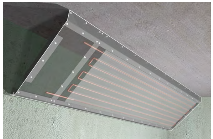
6. Remove 'low-tack' protective covering and clean exposed panel set surfaces.
