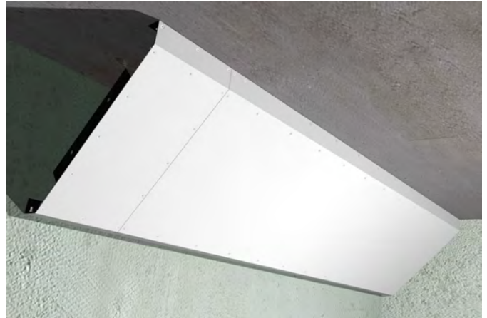
4. Once NOMS Approved Active panel sections are in position make mains connections and install purpose made dummy sections. Use NOMS approved (M6 x 20 Stainless steel countersunk screws) security fixings and suitable thread locking compound.
